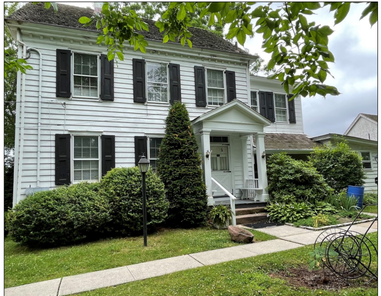
Caldwell Parsonage in Union Township, New Jersey
